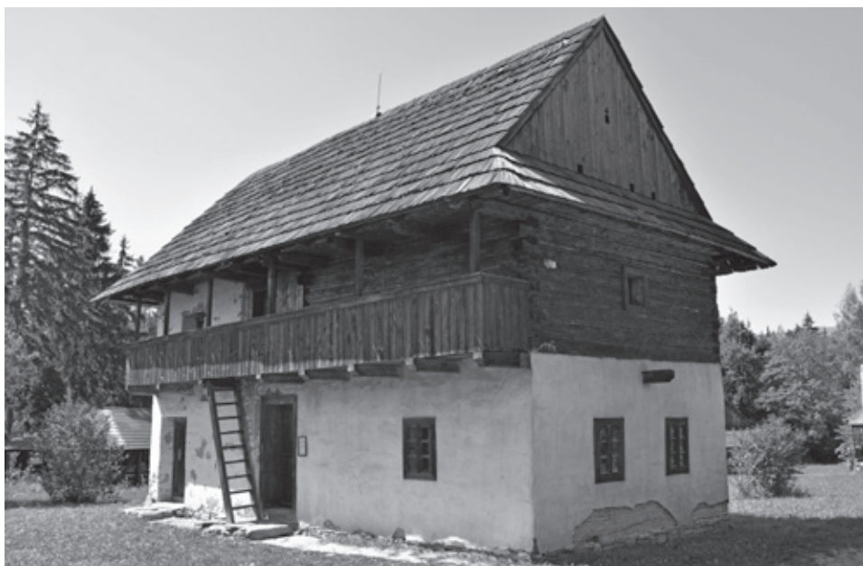
Obr. 8. Poschodový dom z Hornej Breznice č. 140 v Múzeu slovenskej dediny. Foto T. Kadlecová, 2016 Pic. 8. Two-storey house from Horná Breznica no. 140 in the Museum of the Slovak Village. Photograph by T. Kadlecová, 2016
